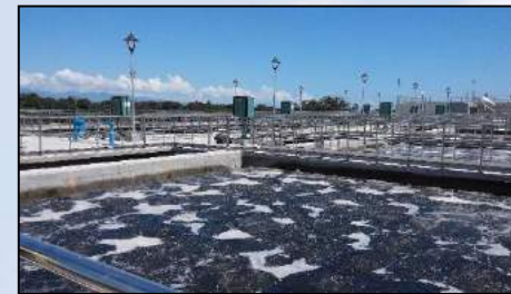
Donggang river 300,000 CMD raw water pretreatment plant
